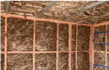
Knauf insulation automatic upgrade to R2.2 in the walls and R3.6 in the ceilings
